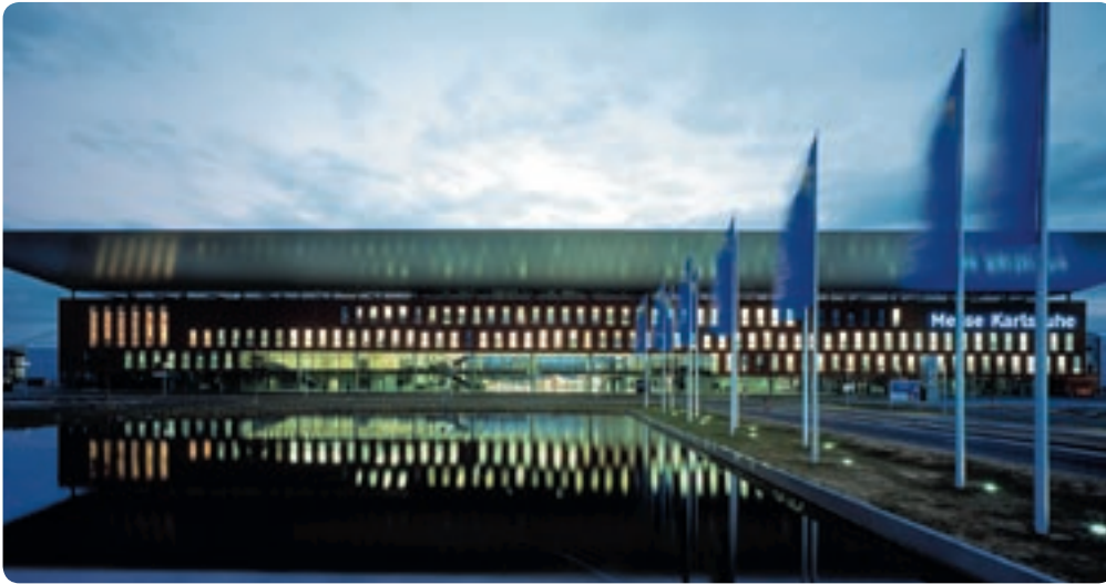
With its new trade fair, Karlsruhe now has an exhibition area of 52,000 square metres
