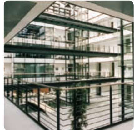
Chemical development and analysis building in Biberach
