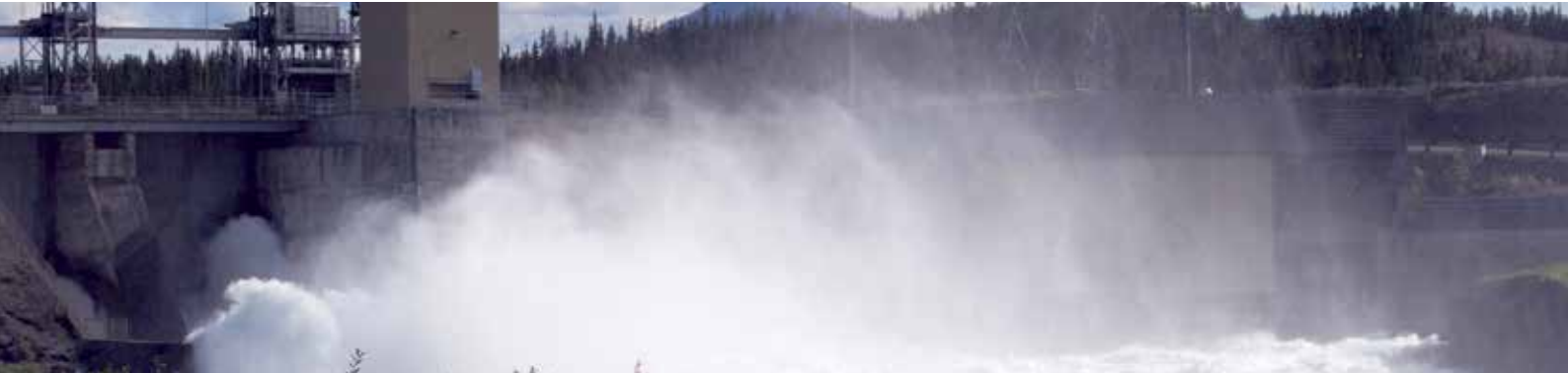
Hydro power plant
